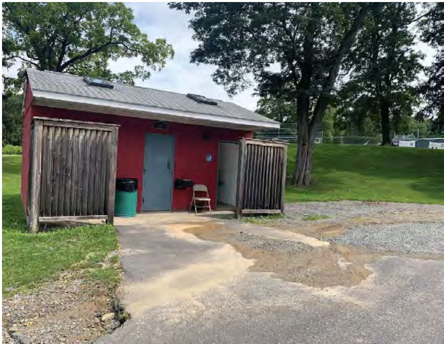
Existing Little League Restrooms
